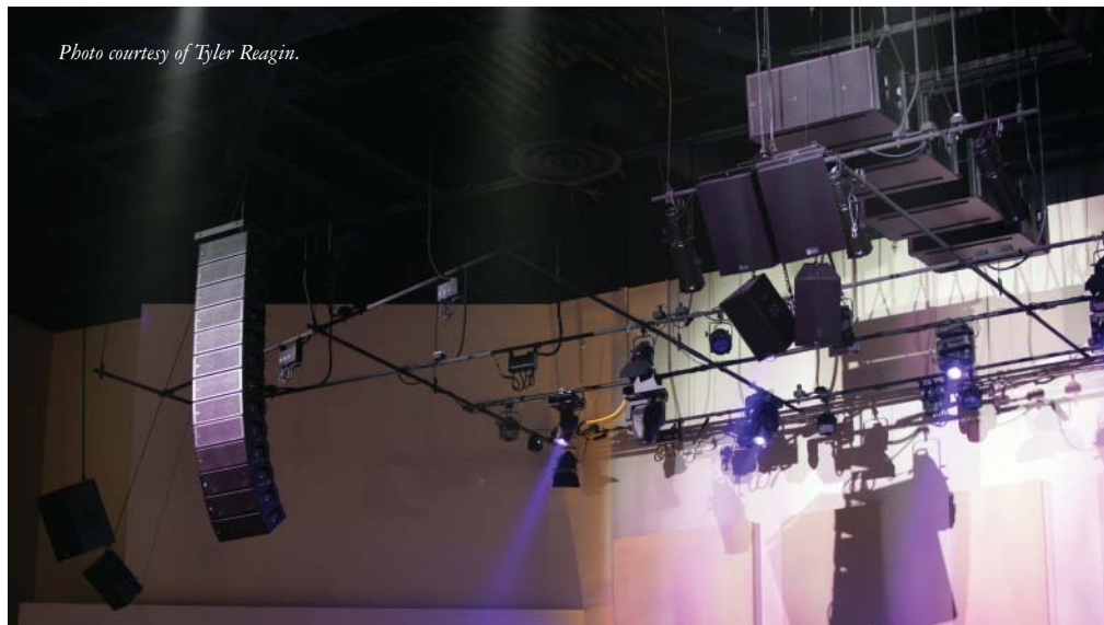
The audio system at Browns Bridge includes Meyer Sound M'elodie line array loudspeakers. There are two primary arrays of 13 cabinets in each array, placed left and right.
